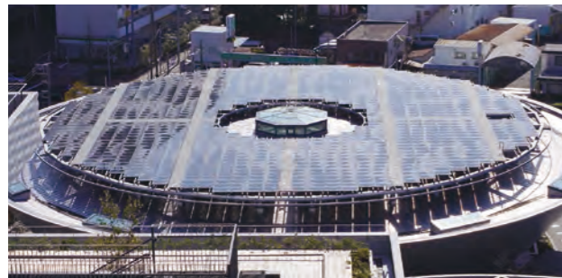
Photovoltaic panels on the rooftop of the forum building within the Haneda Chronogate
